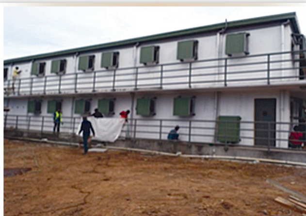
Lautoka Remand Centre - Phase 2
