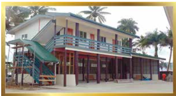
New Transport Shed
